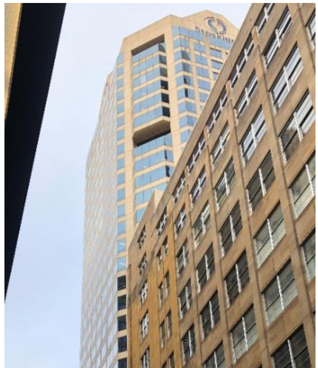
Figure 14 View of top of Piccadilly Tower.
